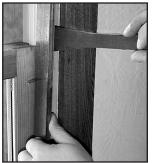
4. Verify the correct fit of the jambliners by placing them against the side jambs. If too tall, cut the bottom of the jambliners in 1/16" increments at a 14° angle. The supplied head jamb gaskets need to be applied to head jamb. Only two are needed - color match to jambliner. Peel off protective backing to expose adhesive and apply gasket to existing head jamb.
