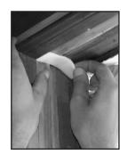
5. The metal clips are to be positioned against the jamb, approximately 4" down from the head jamb and 4" up from the sill. Attach these clips into place using the supplied  $#7 \times 7/8"$ screws. Clips should be installed level and tight to inside stop.
