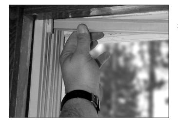
9. When installing the top sash, engage pin in the outside track of the left balance (tilt pin must be above clutch mechanism) then engage the pin in the outside track of the right balance (above clutch mechanism).
