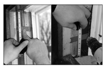
Note: Additional clips are supplied and may be used if required on taller units. Place the additional clips approximately at the midpoint of each sash location if necessary.
